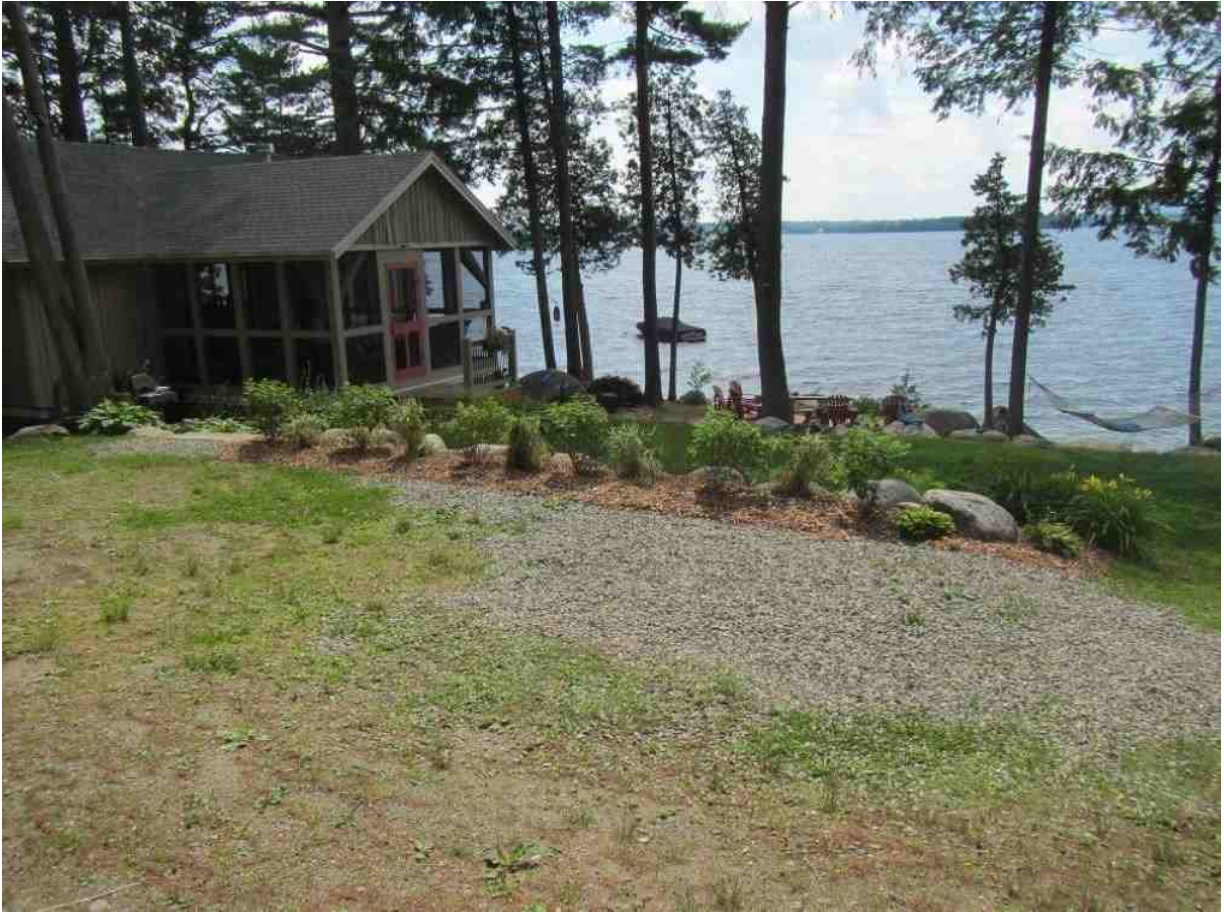
ABOVE: A planted berm at the bottom of a driveway that captures runoff before it reaches the lake. Photo credit: Maine Lakes.
