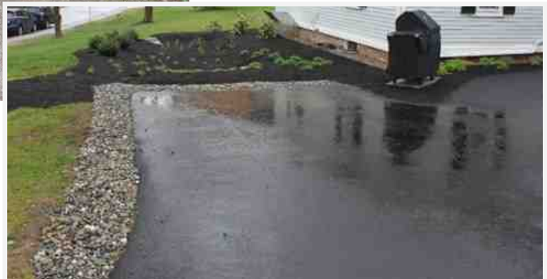
RIGHT: A well-defined parking area surrounded by LakeSmart infiltration practices. Photo credit: SOAK Up the Rain New Hampshire.
