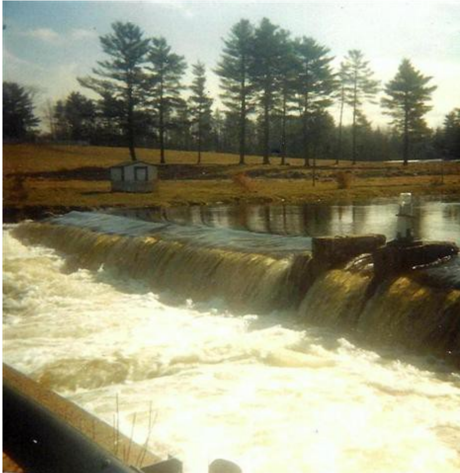
Illustration 3: Now this is a flood. With estimated flows over the dam in excess of 200 cfs, notification of downstream property owners would be warranted! The ponding of the water below the dam indicates that the Clary mill pond dam located just downstream was full and over topping as well. Photograph presumably taken by former dam owner Chester Chase, dated June 1984.
